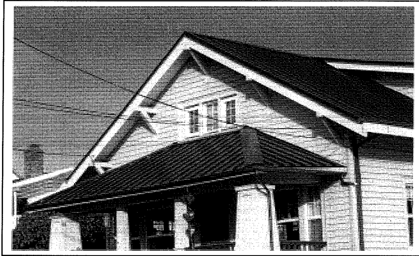
High profile metal seam roof
